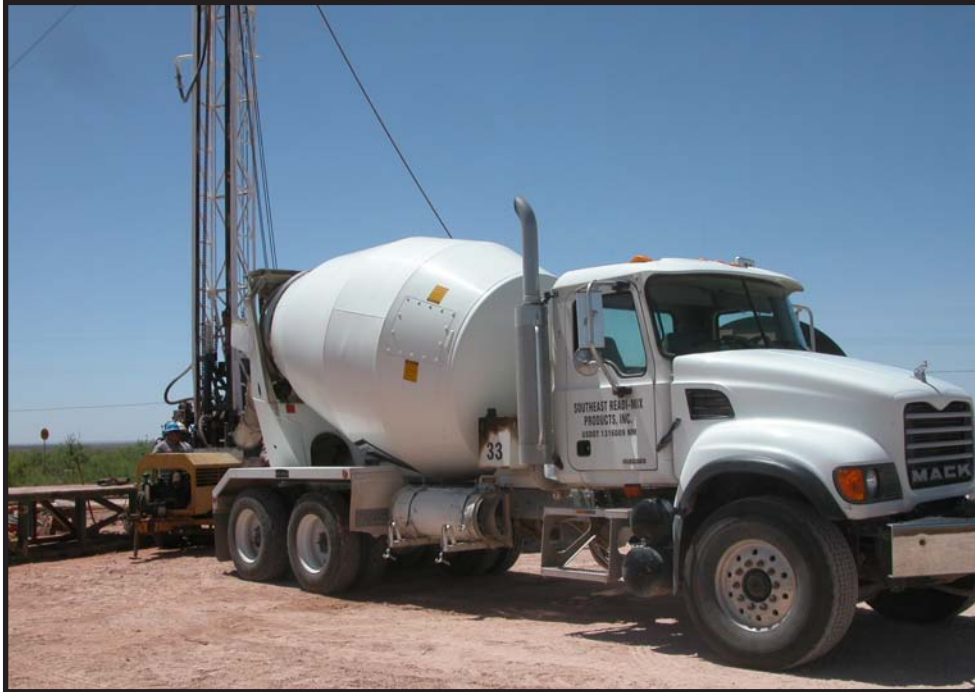
Figure 3-4. Cementing SNL-16 annulus. Cement truck unloading cement into cement pump at SNL-16 to fill annulus above gravel pack and bentonite seal. Photo by Dennis W. Powers.
