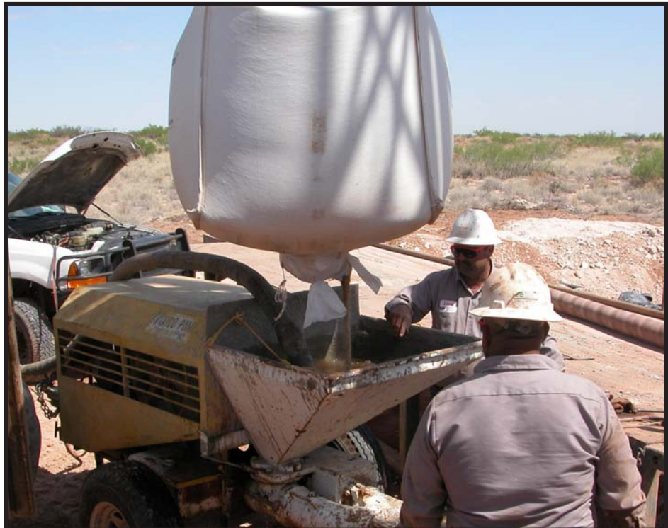
Figure 3-3. Gravel pack for SNL-16. Super sack of 4/10 gravel pumped into SNL-16 behind screened interval. Photo by R.G. Richardson.
